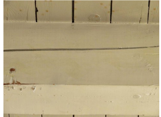
Figure 2 A single wide check on one tangential surface of a timber
