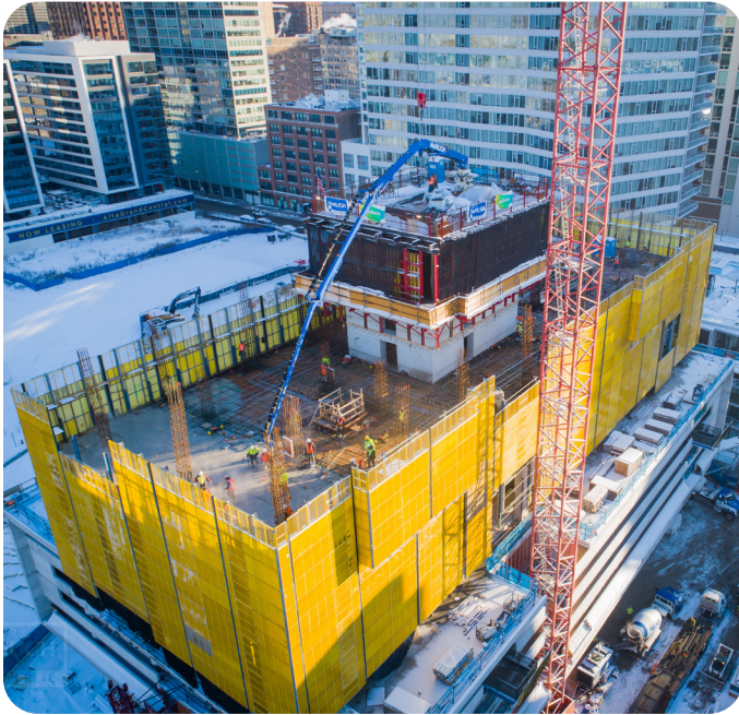
The Reed at Southbank under construction.
