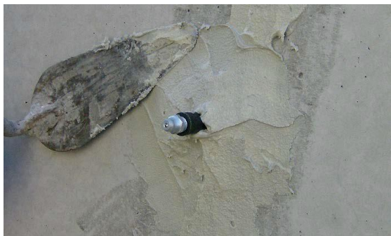
Figure 2. Sealing the surface mounted nipples by using MasterFlux® ANC 920 SF
