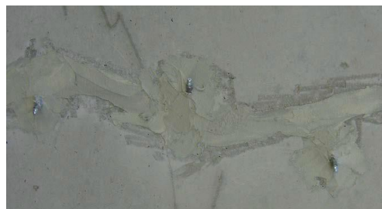
Figure 1. Socket type nipples placed around the crack and sealed with proper epoxy adhesive from MasterStrength™ series.
