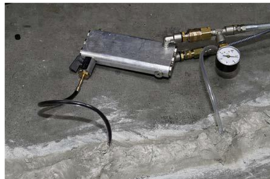
Figure 3. Injecting MasterFill™ ER 1380 by using a 2C pump to repair a concrete floor.
