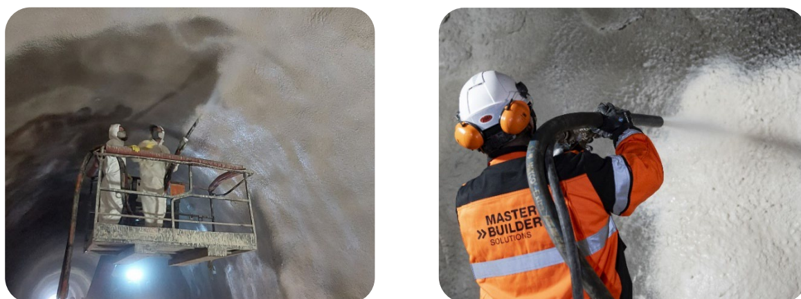
Photos 15 : Application manuelle
