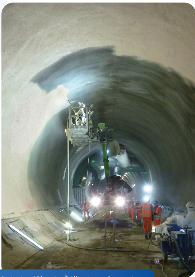
Application of MasterSeal® 345 waterproofing membrane
