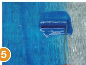
5 Apply second coat of MBrace Saturant
