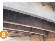
6 Position MBrace Laminate and apply to substrate
