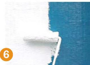
6 Apply MBrace Topcoat (optional)
