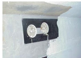
More tensile pull off tests showing complete break in concrete substrate. These tests are performed on a sacrificial test piece of FRP laminate
