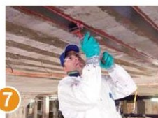
5 Apply MBrace Laminate Adhesive to Laminate
