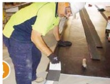
4 Remove Peel-Ply from laminate. The easiest way to take off the peel-ply is with a cutter/Stanley knife. Start to lift the peel-ply with the knife (start from the corner as it will be the easiest spot) and move the knife across the sheet. Once the peel-ply has started to lift, pull back by hand the required length of the Laminate.
