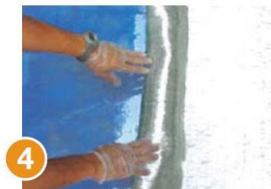
4 Apply MBrace Fibre Reinforcement
