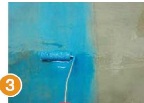
3 Apply first coat of MBrace Saturant
