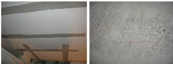
Localized surface preparation of concrete ready to receive MasterBrace®Laminate system
