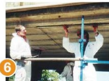
3 Apply MBrace Laminate Adhesive to substrate
