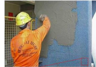
Cementitious coating being applied over an FRP system
