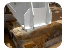
• Before grouting, flood the formwork area with water to check for leaks. Address any leaks identified before proceeding with grout placement.
