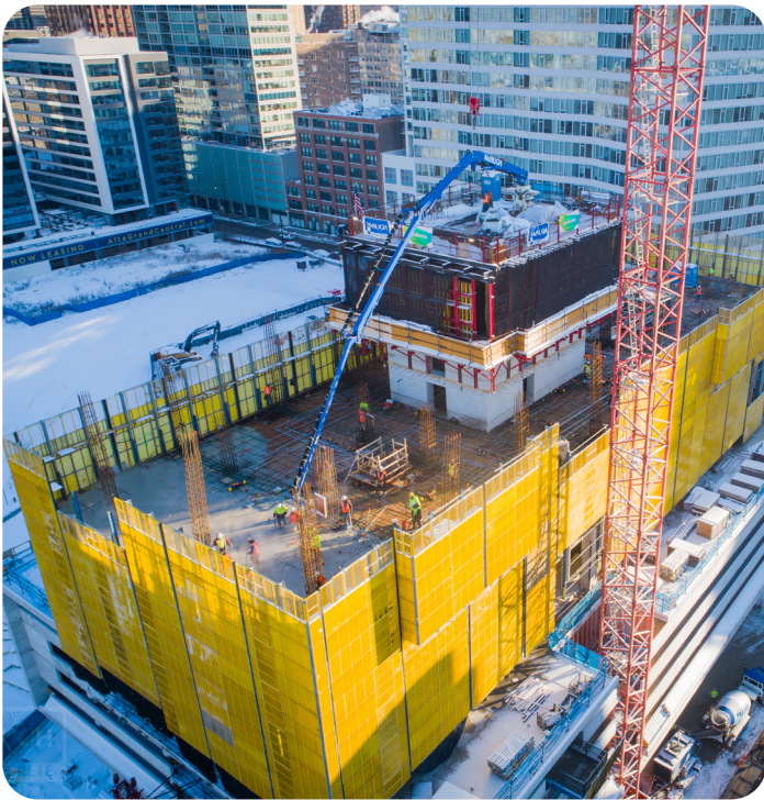
The Reed at Southbank under construction.
