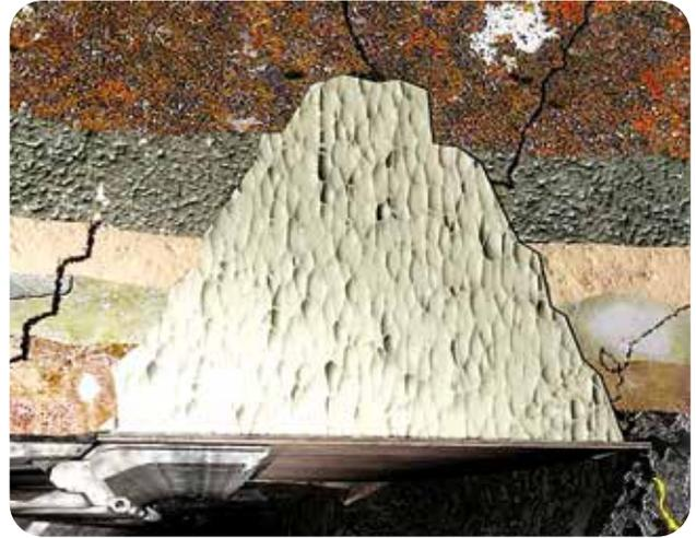
Cavity filling with MasterRoc® MP 367 Foam
