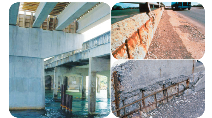
The bridge on the right is experiencing heavy corrosion. The bridge on the left was built to prevent corrosion by using high performance concrete with durability-enhancing admixtures. Durability issues, such as corrosion of reinforcing steel in roads, bridges, and parking structures, can be effectively addressed with durability-enhancing admixtures from Master Builders Solutions.
