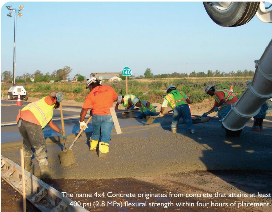
The name 4x4 Concrete originates from concrete that attains at least 400 psi (2.8 MPa) flexural strength within four hours of placement.
