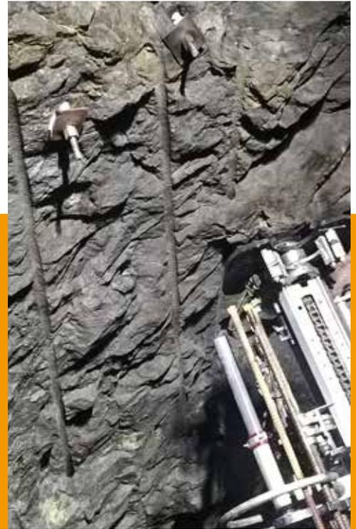
Self-drilling anchor with MasterRoc RBA 380
