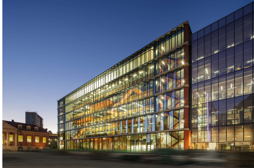
The Braggs Building, University of Adelaide
