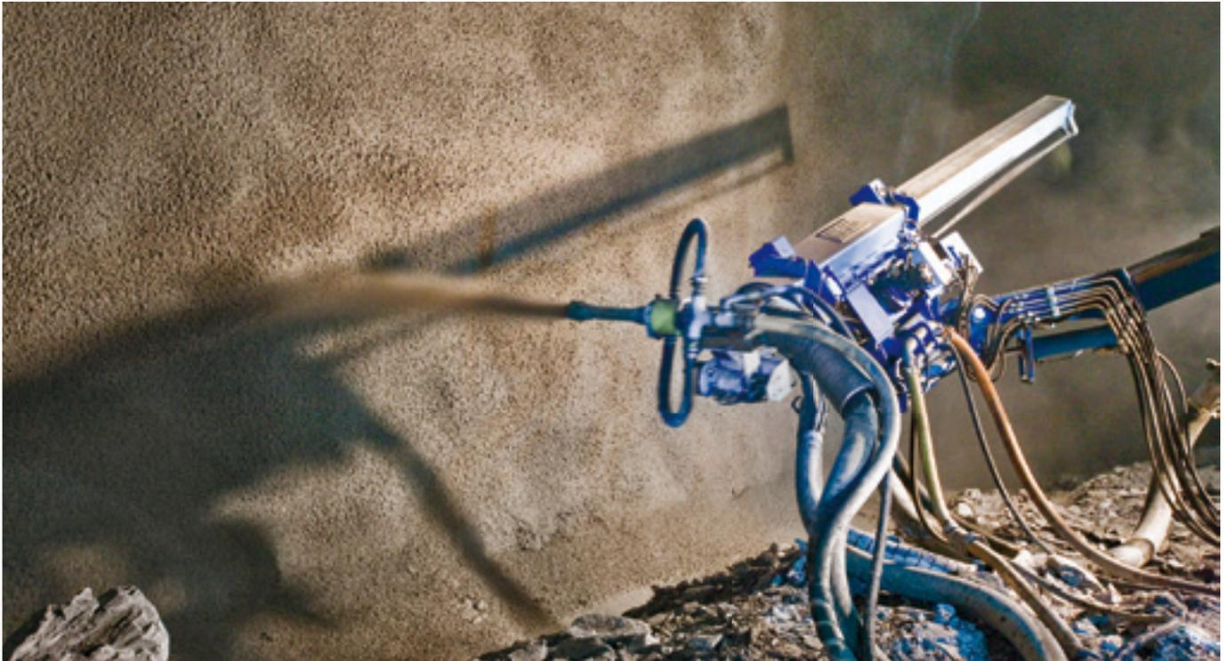
Sprayed concrete technology has revolutionized tunnel construction and mining operations since the middle of the 20th century. The development of material science and performance together with advances in spraying equipment technology have made sprayed concrete the building material of choice for today's underground construction projects.
