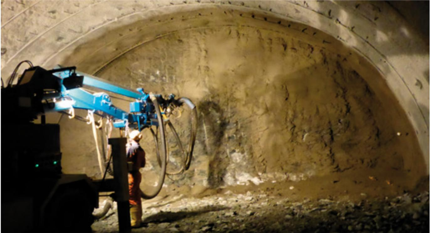
Sprayed concrete applications must ensure safety and be formulated to last. Master Builders Solutions offers a wide range of admixtures for addition during concrete batching and on-site.
