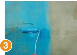
3 Apply first coat of MBrace Saturant
