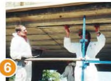
3 Apply MBrace Laminate Adhesive to substrate
