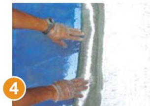
4 Apply MBrace Fibre Reinforcement
