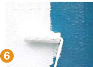
6 Apply MBrace Topcoat (optional)
