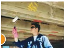
1 Apply MBrace Primer onto prepared concrete substrate (optional)
