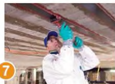
5 Apply MBrace Laminate Adhesive to Laminate
