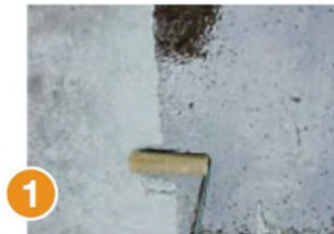
1 Apply MBrace Primer onto prepared concrete substrate (optional)
