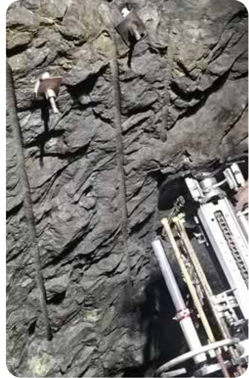
Self-drilling anchor with MasterRoc® RBA 380
