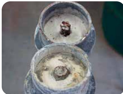
With corrosion inhibitor
