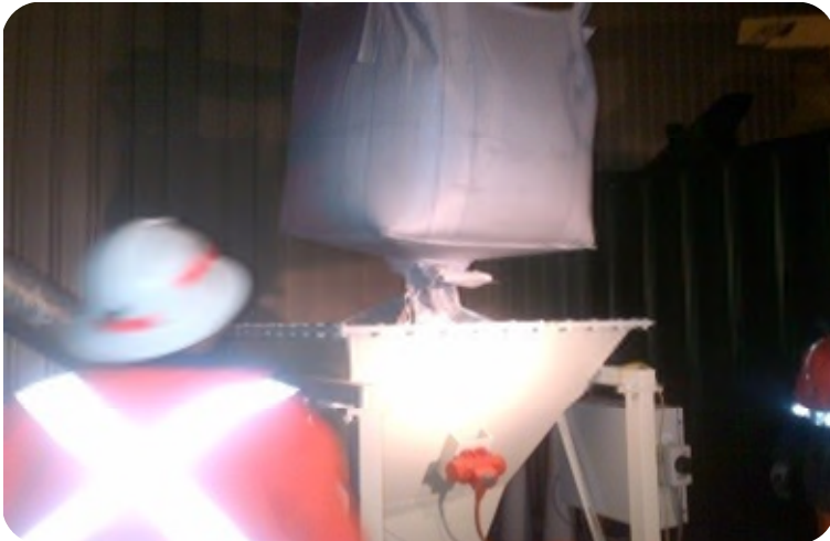
Bulk bag loading into auger hopper for transfer into concrete agitator
