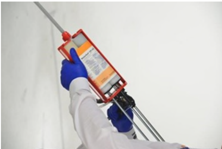
Figure 14 - Withdraw plunger by releasing the catch plate and remove the cartridge from the gun.
