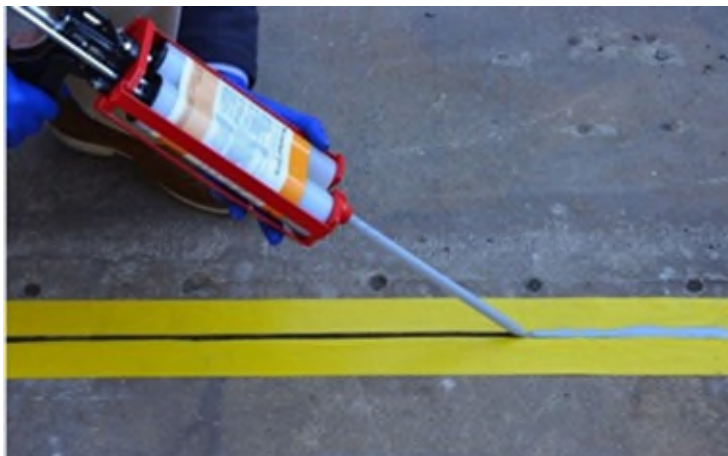
Figure 10 - Gun material into the joint with smooth presses of the trigger to fill the joint.
