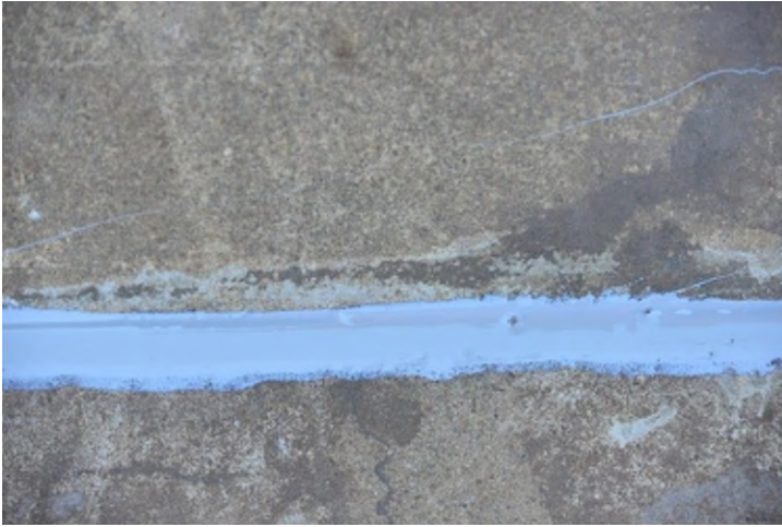
Figure 13 - Leave joint to cure and return to service after 1 hour
