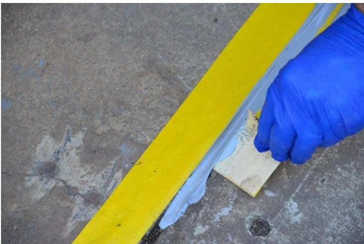
Figure 12 - Remove tape as soon as tooling is complete
