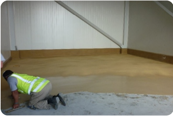
Installing Ucrete DP floor in newly expanded Takanini Plant
