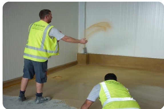
Applying the non-slip aggregate
