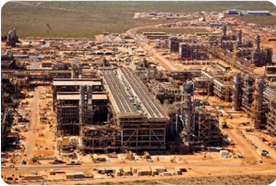
The Gorgon project under construction
