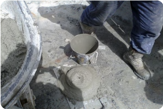
180mm slump shotcrete at 24 hours age
