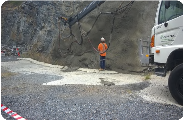
Applying shotcrete at the Legacy Way spoil tunnel portal
