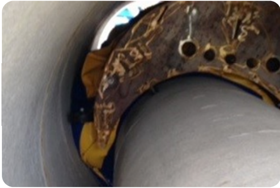
Mock-up inflatable bags before filling with precision grout
