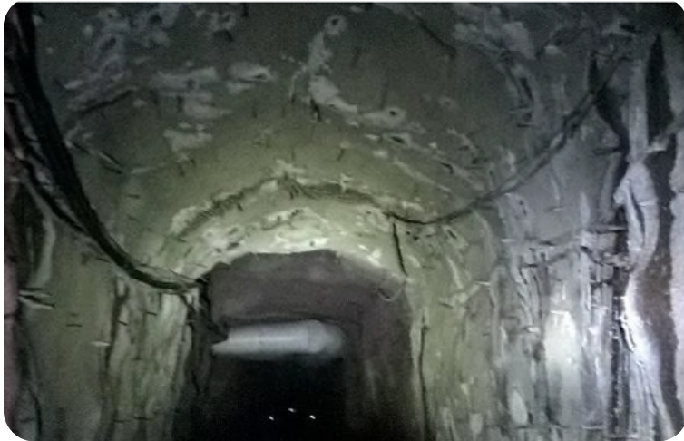
An image showing the drive with MasterLife 300D in the shotcrete
