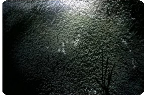
Shotcrete with the MasterLife 300D included
