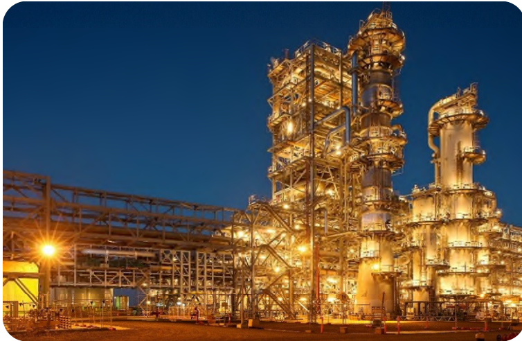
The Pluto facility in Western Australia. Image source: Woodside image gallery
