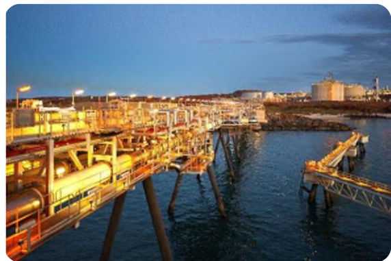
Loading jetty at Pluto LNG onshore gas plant. Source: Woodside image gallery
