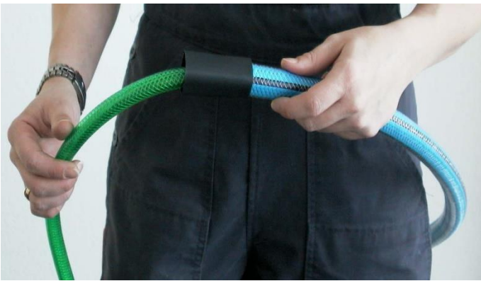
Figure 8: Place the shrink sleeve over the join
