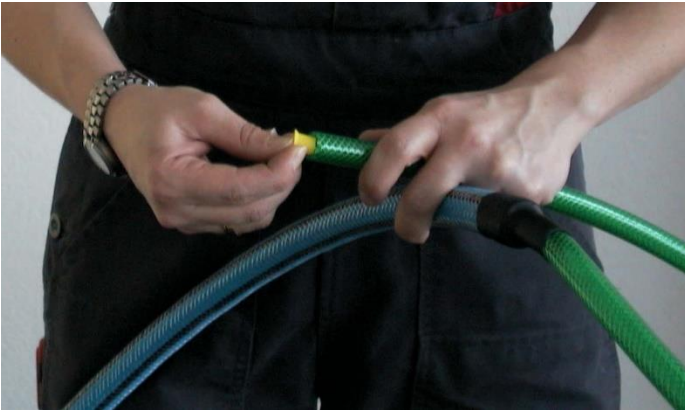
Figure 11: Cap the ends to prevent blockage prior to installation
