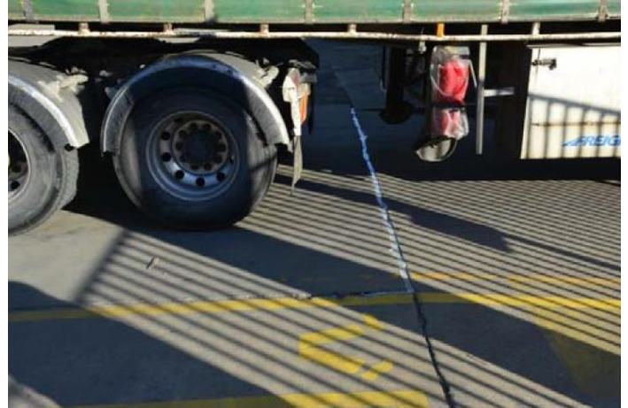
Traffic moved over the joint within 15 minutes of application
