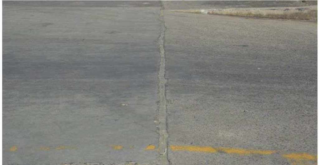
The repaired joint outside MB Solutions Seven Hills warehouse driveway
