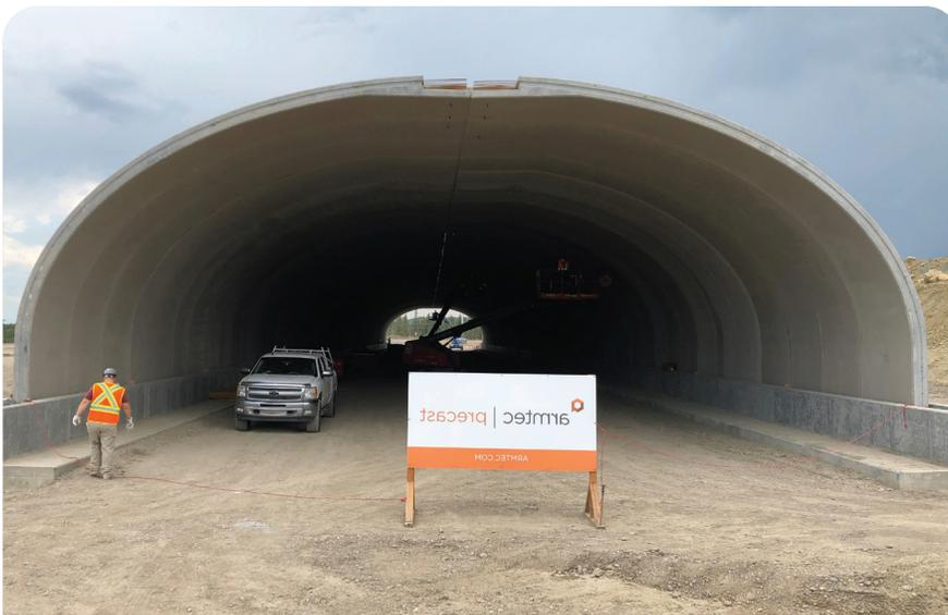
BEBO<sup>®</sup> Arch Systems are reinforced precast concrete arch structures that are covered with a membrane and overfilled with earth to form a bridge, tunnel or other hollow structure. The Southwest Calgary Ring Road (SWCRR) highway tunnel, located in Calgary, Alberta, Canada, will be the longest BEBO structure in Canada, measuring 1 655.5 m (543 ft).
