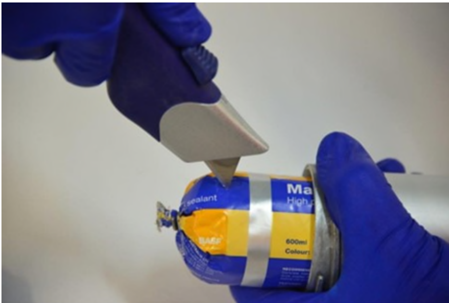
Figure 8 - Cut a vertical slit in the sausage about 25mm long. It is not necessary to remove the top of the sausage for the sealant to be extruded properly.
