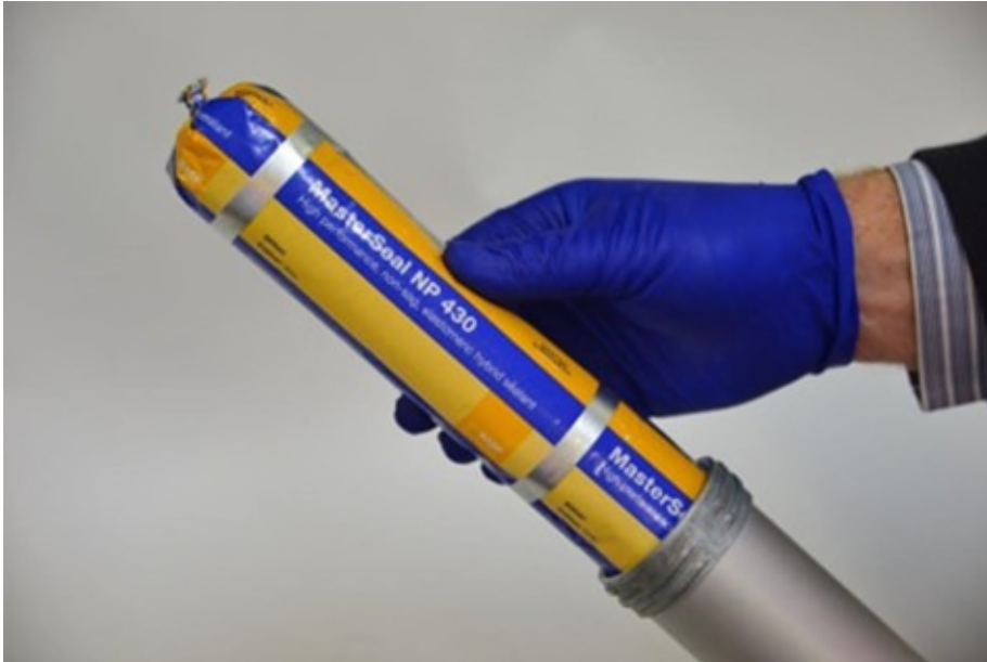
Figure 7 - Insert sausage into the gun until only the top is sticking out.
