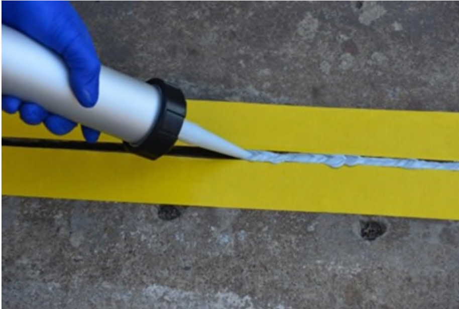
Figure 11 - Insert the nozzle into the prepared joint and with the nozzle just touching the backer rod squeeze out the sealant allowing it to extrude around the nozzle and draw the nozzle back along the joint whilst gently continually extruding the sealant.
