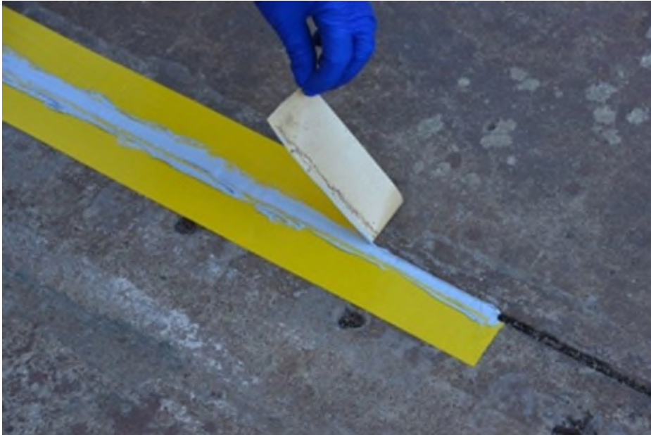
Figure 13 - Remove the protective tape from the sides of the joint before the sealant skins.
