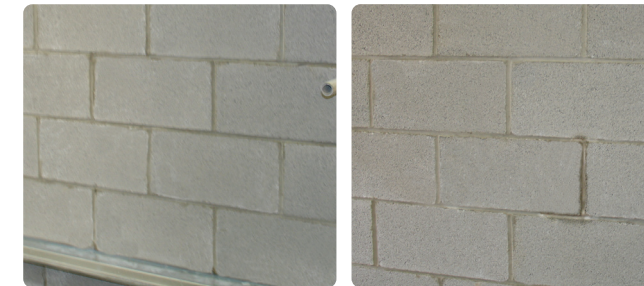
Project # 05-281 - Initial Testing MasterPel 240-Treated Wall
