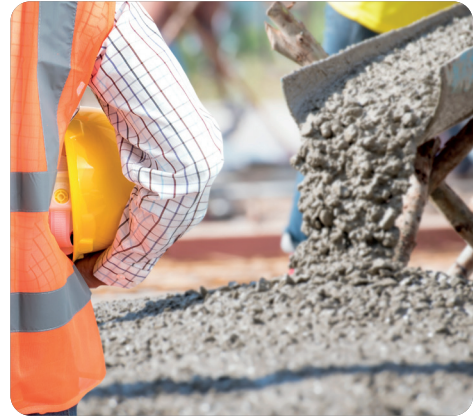
Leading edge concrete reinforcement
