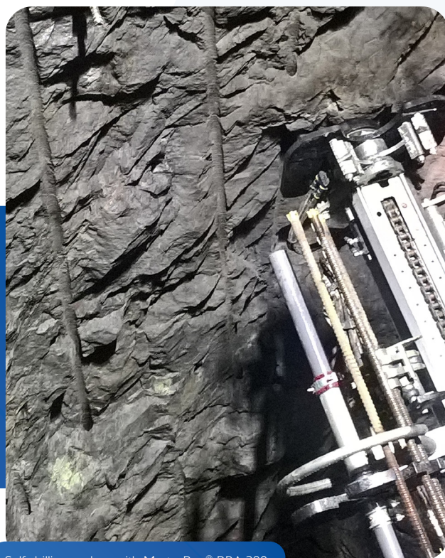
Self-drilling anchor with MasterRoc® RBA 380
