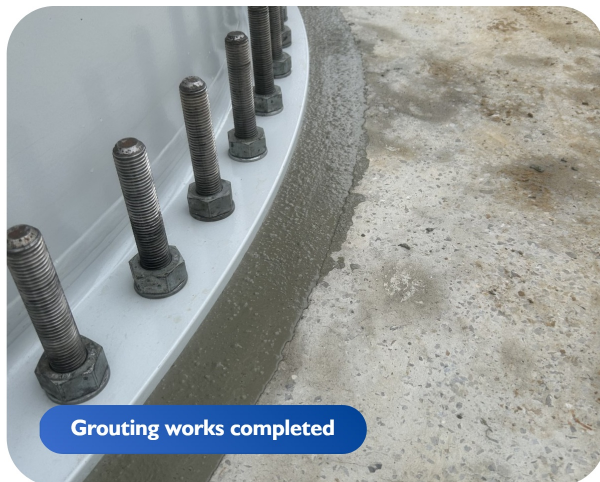
Grouting of tower flange
