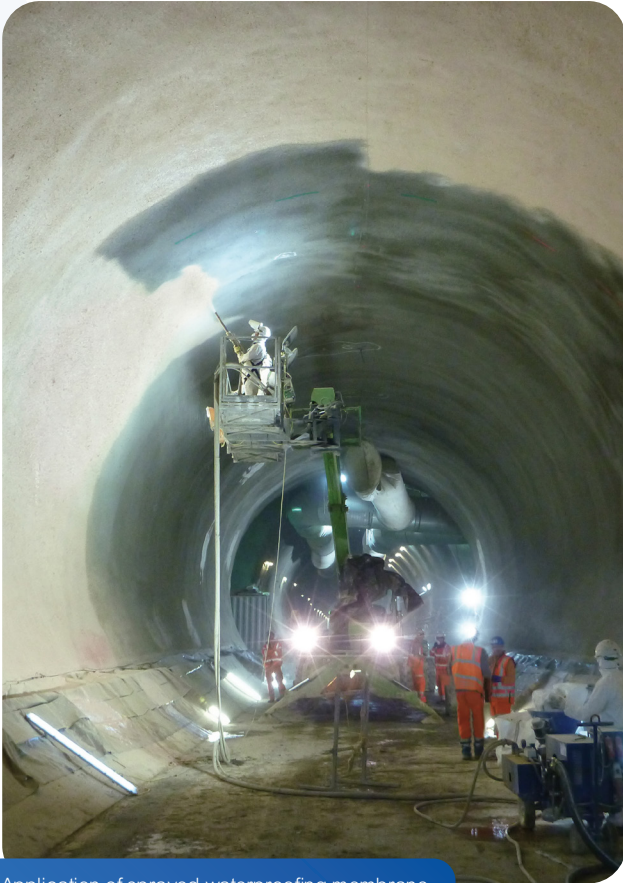
Application of sprayed waterproofing membrane
