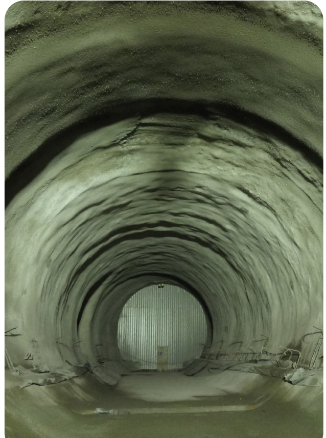
Permanent sprayed concrete lining with sprayed waterproofing membrane
