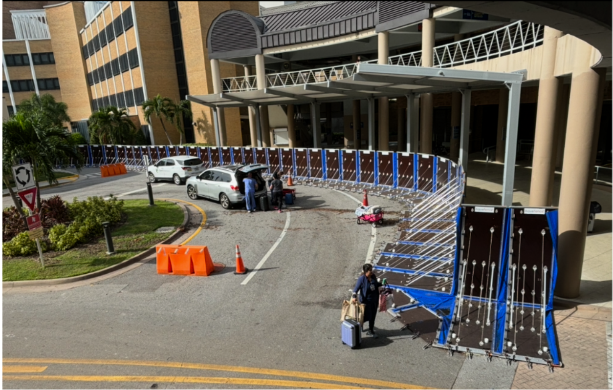
Figure 3. Mobile flood barriers at Tampa General Hospital. Photo courtesy of “Hurricane” Hal Needham.
