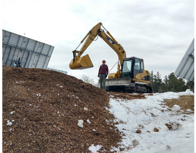
First test pile for snow depot 2018
