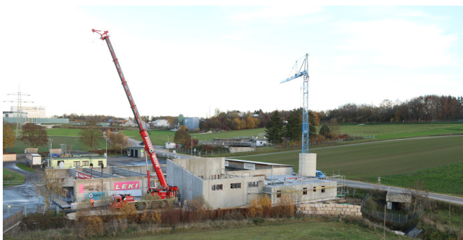
Drone Shot of Construction Site
