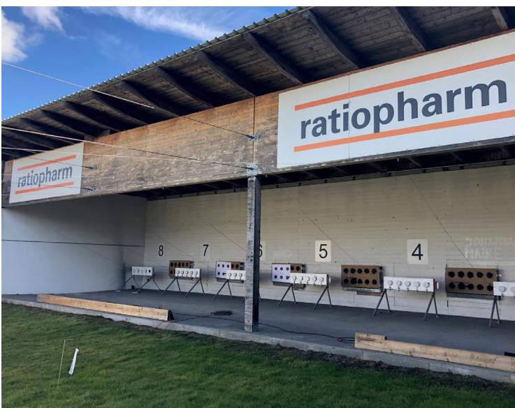
Roofed shooting range
