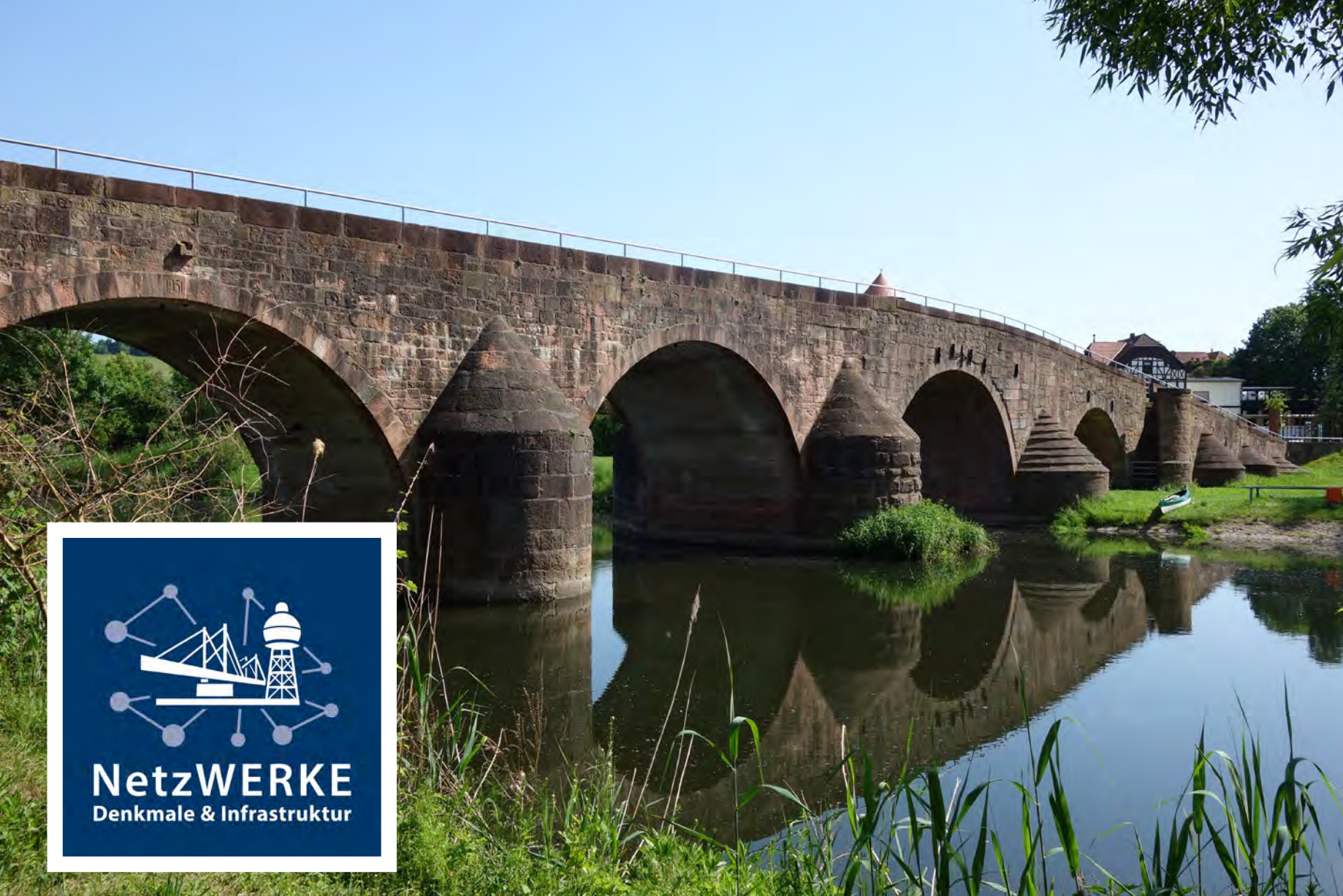
Werrabrücke Vacha, © Michael Höhn
