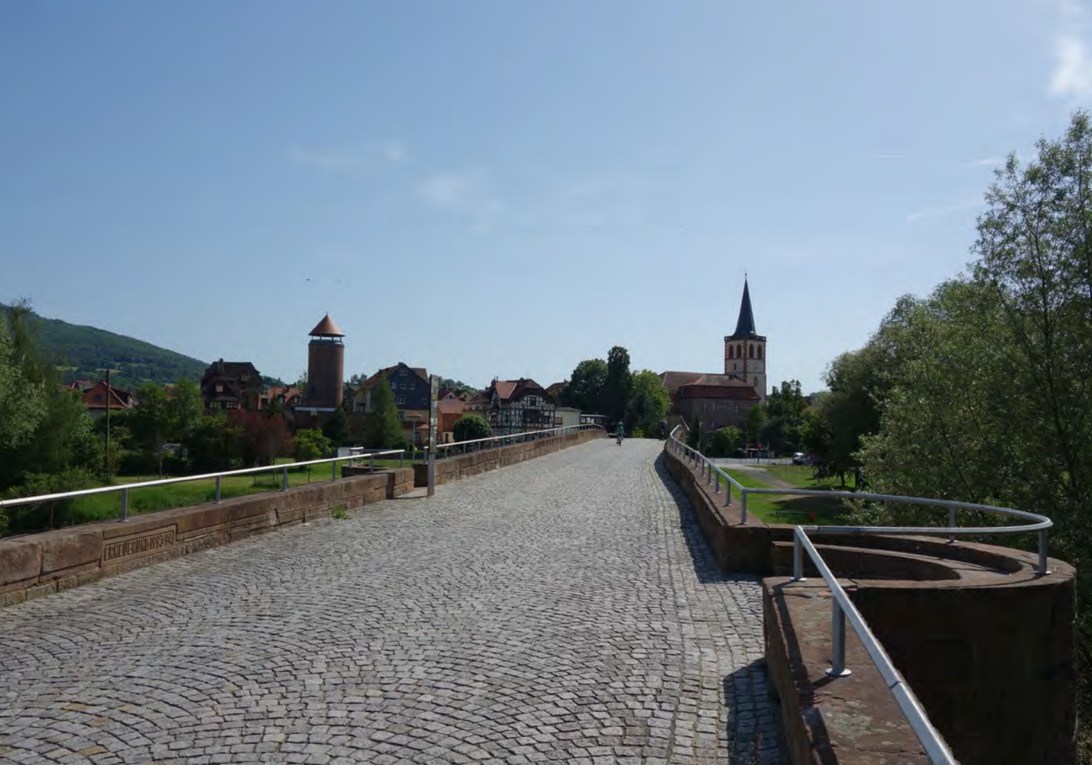
Werrabrücke, Vacha, © Michael Höhn
