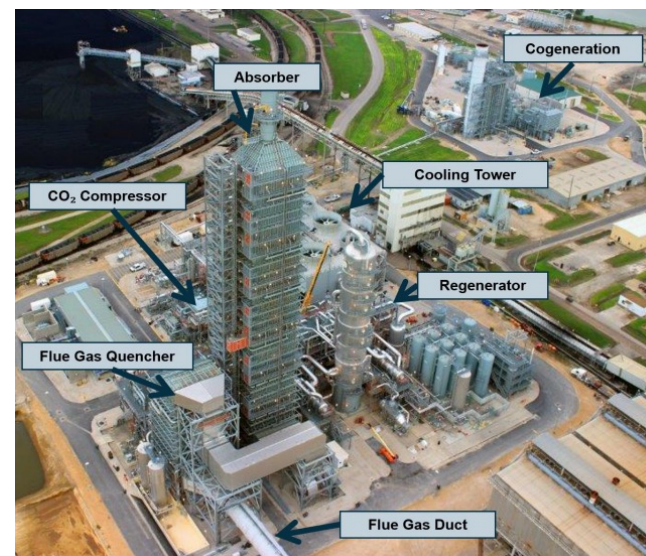
MHI Design (Steel) : 36m (H) DCC / 110m (H) Absorber/ (4700 tCO 2 /d)
