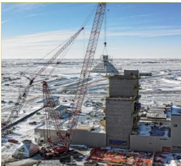
Shell Cansolv Design (Concrete): 11m x 11m (W) x 19 (H) DCC 11m x 11m (W) x 54m (H) Absorber / (3000 tCO 2 /d)
