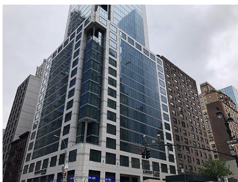
Source: Site Inspection.
