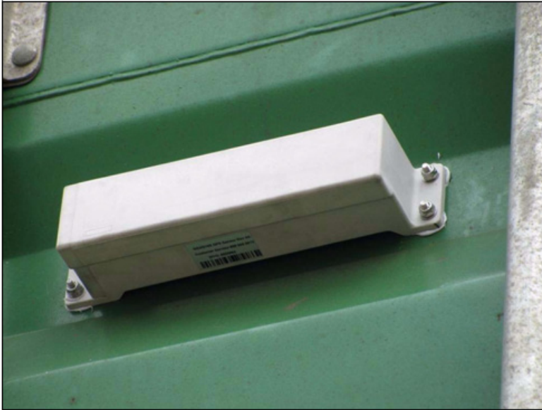
Figure 9 - Proper orientation with label facing downwards
