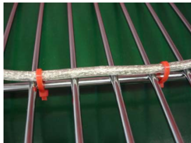
Figure 3-5: Example of Cable Stress Relief
