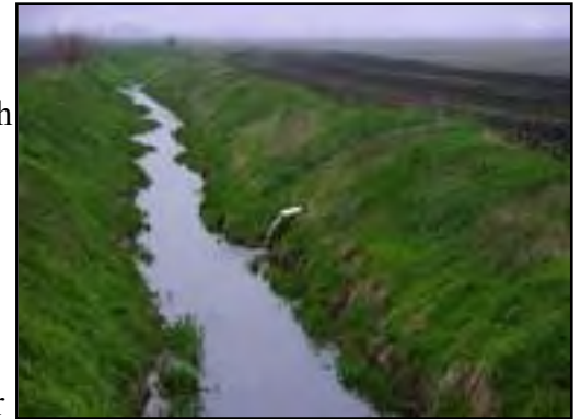
Figure 44: Photo of tile drainage on an agricultural field (Royer, 2010)
