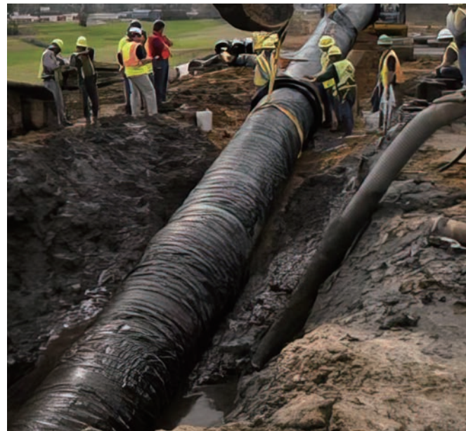
Figure 1: HDD cartridge method with Ductile iron pipe
