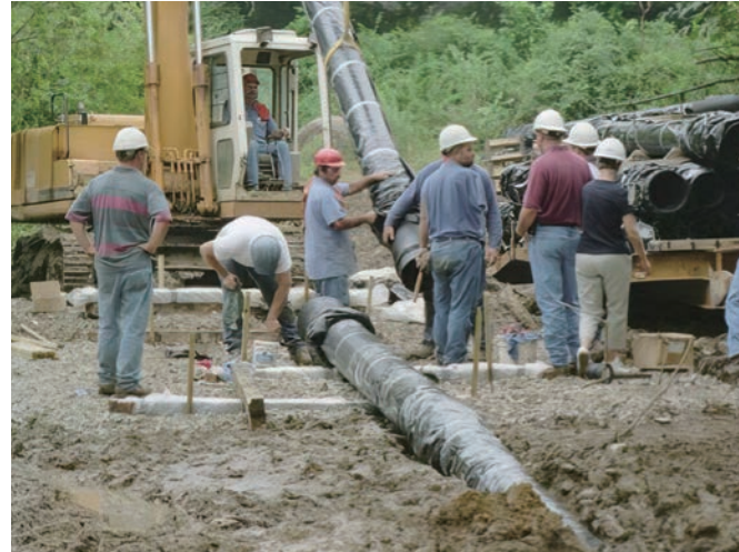
Figure 9: Cartridge method with Ductile iron pipe
