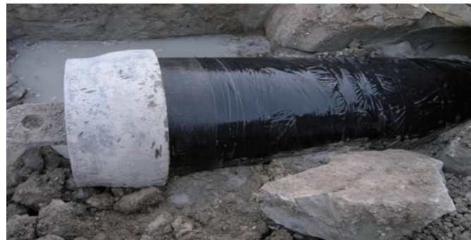
Figure 19: Exposed polyethylene encasement after HDD installation—Polyethylene encasement uncompromised from installation
