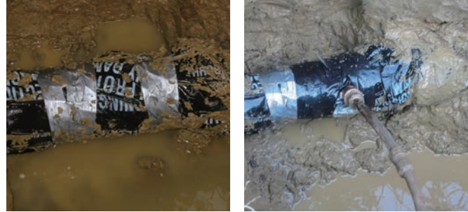
Figure 17: Polyethylene inspection and tapping on Ductile Iron pipe
