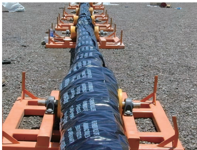
Figure 2: HDD assembled-line method with Ductile iron pipe
