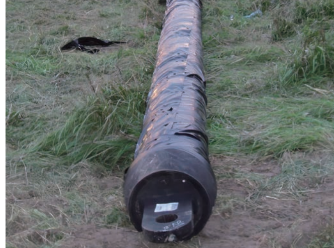
Figure 15: Pulling head attached to polyethylene encased Ductile iron pipe
