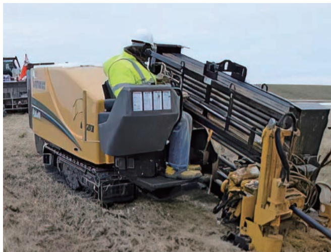
Figure 4: HDD boring machine - courtesy of Trenchless Technology Magazine
