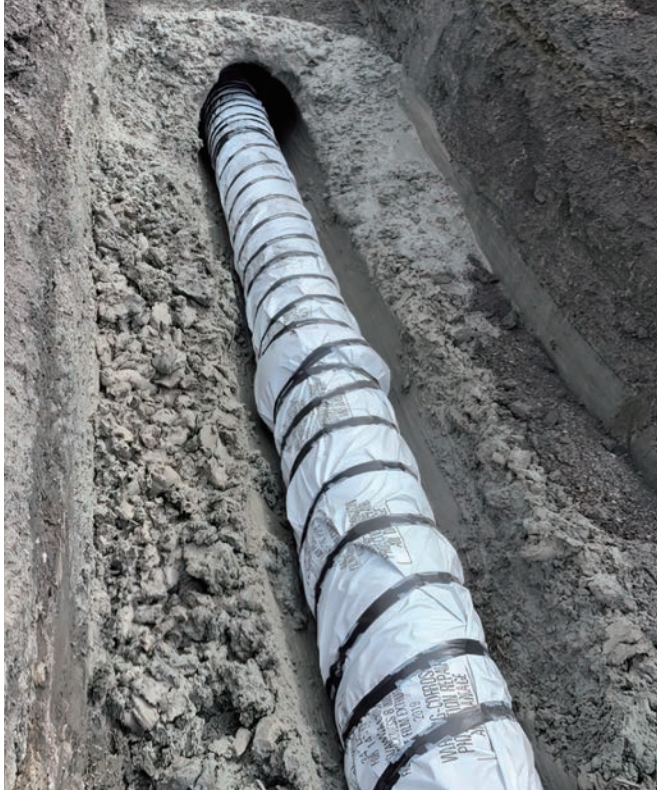
Figure 16: Spiral installation of V-Bio® enhanced polyethylene encasement on Ductile iron pipe
