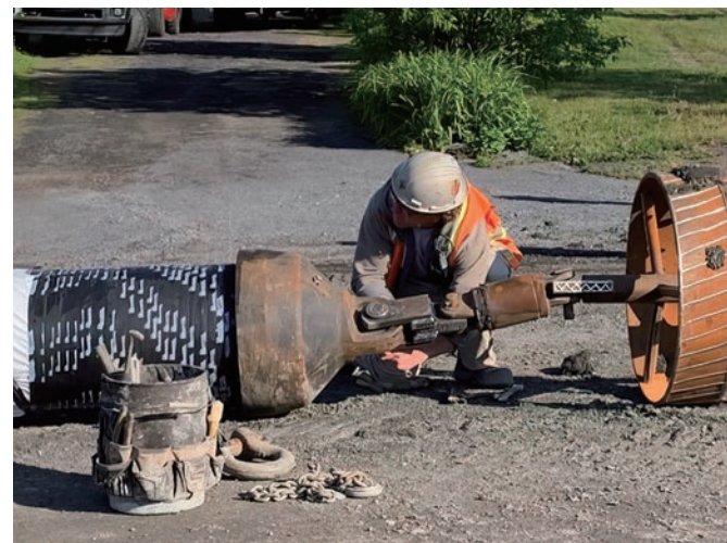
Figure 5: Attaching back reamer and swivel connection to Ductile iron pipe
