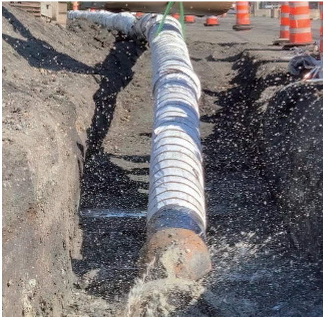
Figure 6: Ductile iron pipe pullback — entering the bore path
