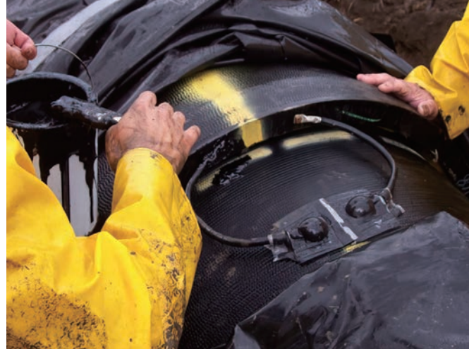
Figure 20: HDD Installation using bonded joints
