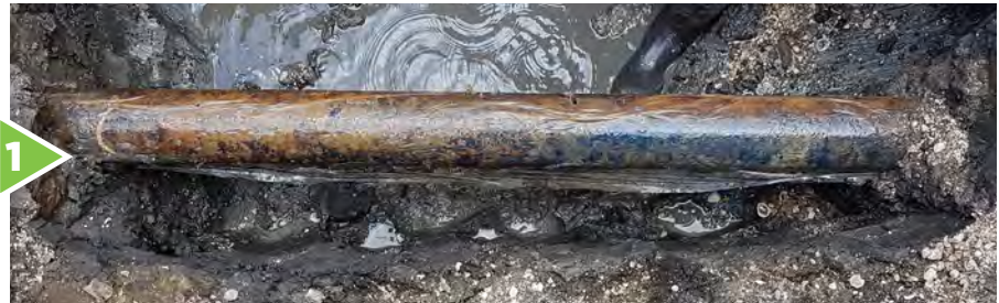
Polyethylene Encasement prior to removal.
