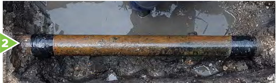
Polyethylene Encasement has been removed.
