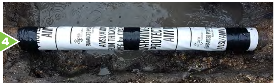
Pipe rewrapped with Polyethylene Encasement
