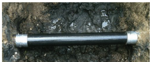
Pipe after cleaning
