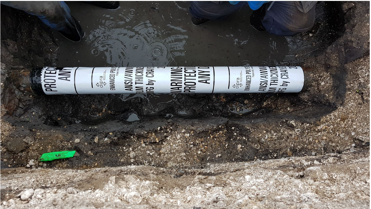
G: Pipe encased in V-Bio ® enhanced polyethylene encasement prior to backfilling
