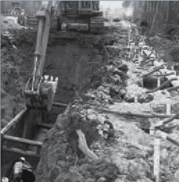
Well-suited for difficult installations due to its inherent strength, Ductile Iron is an excellent piping material for use in gravity sewer applications. Its superior ring strength, combined with its bottle-tight joints, makes it ideally suited for deep trenches and installations in areas of high water table.
