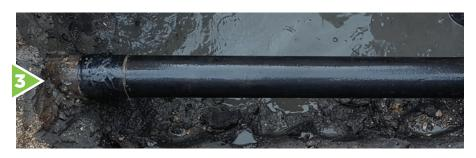
Pipe rewrapped with polyethylene encasement
